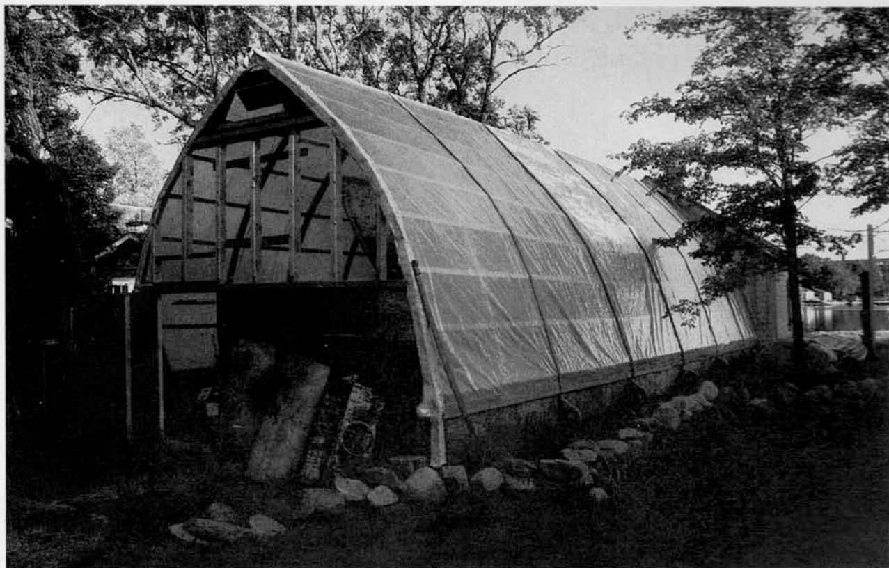
The author's bowed-frame temporary boat shed attached to the back of his workshop. The bowed rafters allow the width of the building to be carried higher than that of an A-frame structure.
